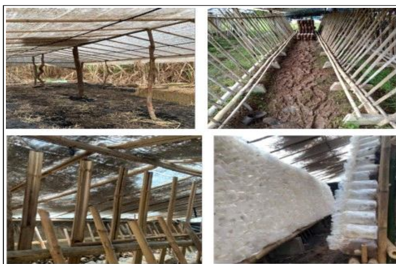
Fig 1: Design and installation of the house structure.
